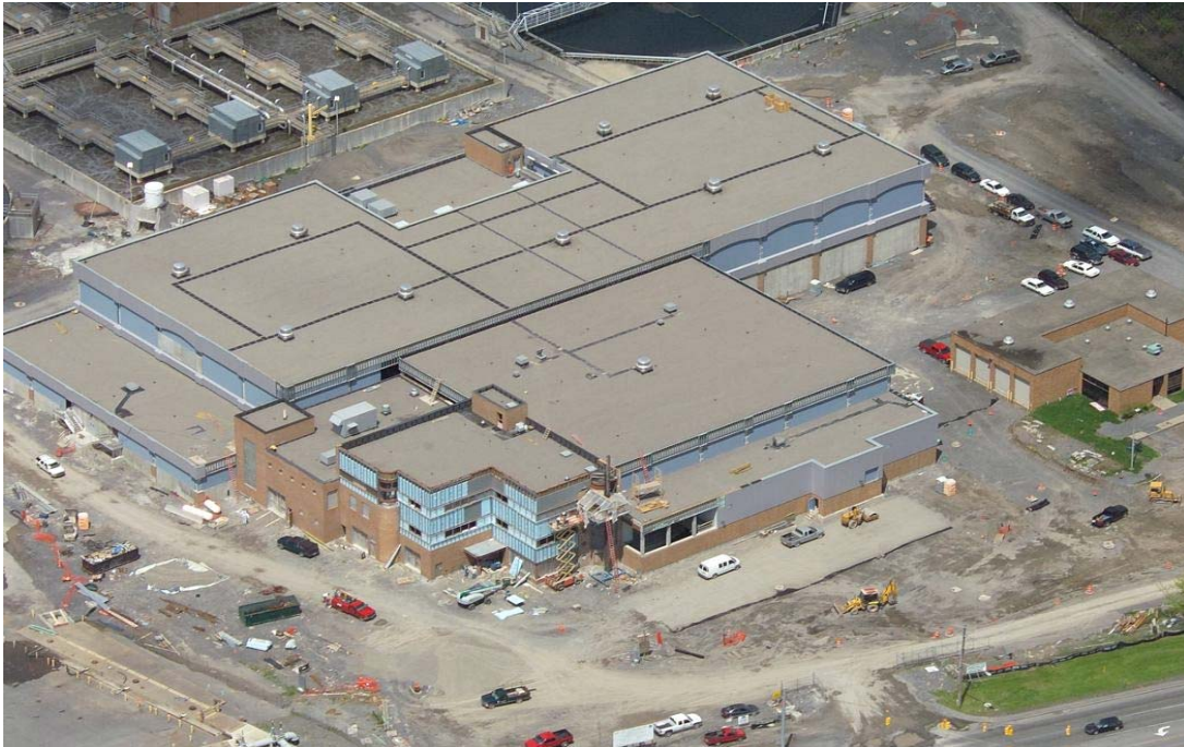
New Metro Complex at the 90% Completion Point
