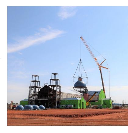
engineering, construction, and architecture. Early on, construction teams made the decision to build the dome on the ground on concrete piers rather than 100+ feet in the air. This increased safety on the jobsite and eliminated the need for scaffolding, lifting equipment, and extra labor hours needed to build above ground — and it was easier to lift it for final placement.
