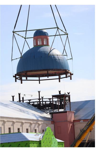
"It starts with getting the dimensions and details of what is being lifted," Rivers says. "We start developing where the lifting-load attachment was going to be, the lifting weight, the rigging components, and the capacity of the crane."
