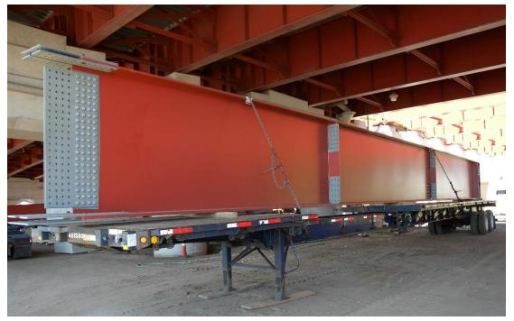
The delivery sequence and location for receiving steel at a project site is determined by the available laydown and shakeout space. Typically, steel is delivered at the project site first in the morning and then after lunch. Projects with a staging area allow shakeout and positioning for more efficient erection. These two factors create significant constraints for plans.
