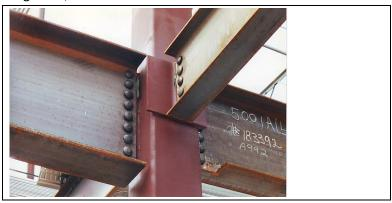
Shear connections, the most common type for structural steel members, transmit shear from one steel member to another. They are not able to resist moments at the connections, and therefore allow rotation at the connection under lateral loading.
