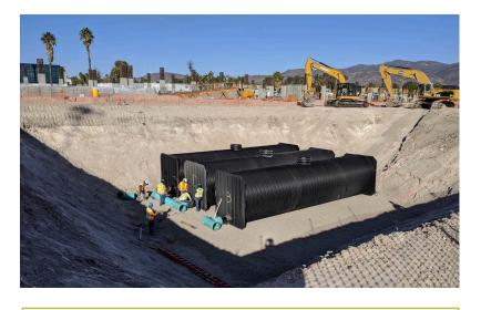
Installation of below-grade stormwater storage - stored water will be used to irrigate the landscape as needed
